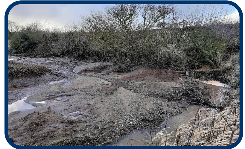
Figure 1. Re-profiled bend after two months
